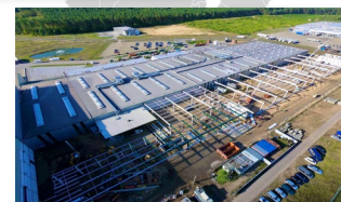
MMP Expansion Poland
