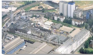
MM Neuss Rebuild (Liner)
