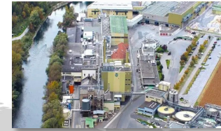
MM Frohnleiten Rebuild (CRB)
